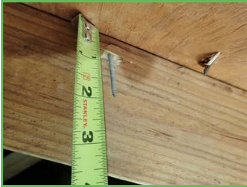
Roof Deck Attachment
