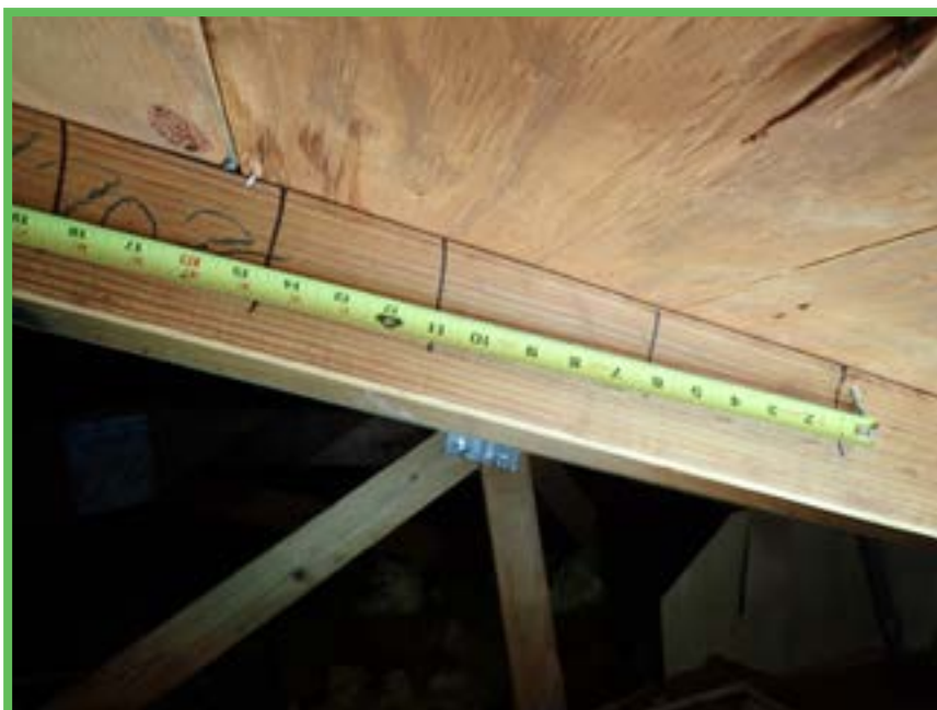
Roof Deck Attachment
