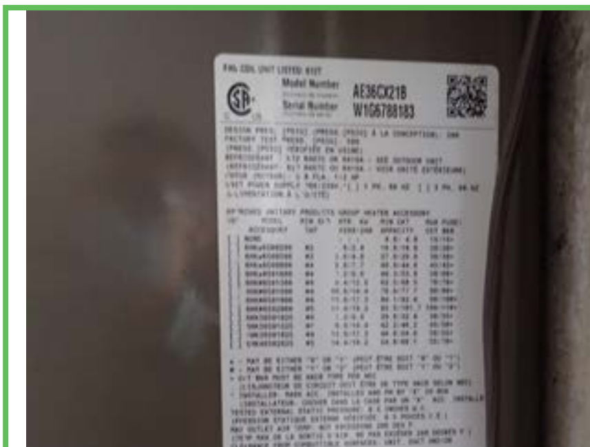
HVAC Air Handler Data Plate
