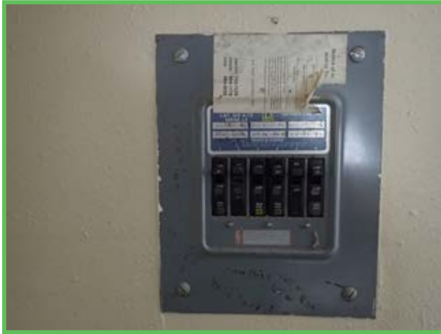
Electric SubPanel
