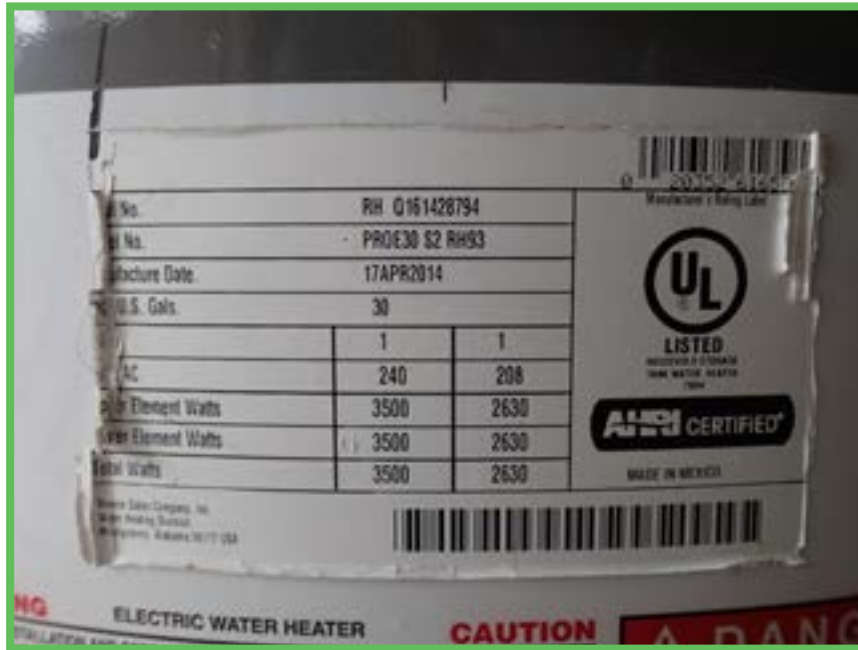
Water Heater Data Plate
