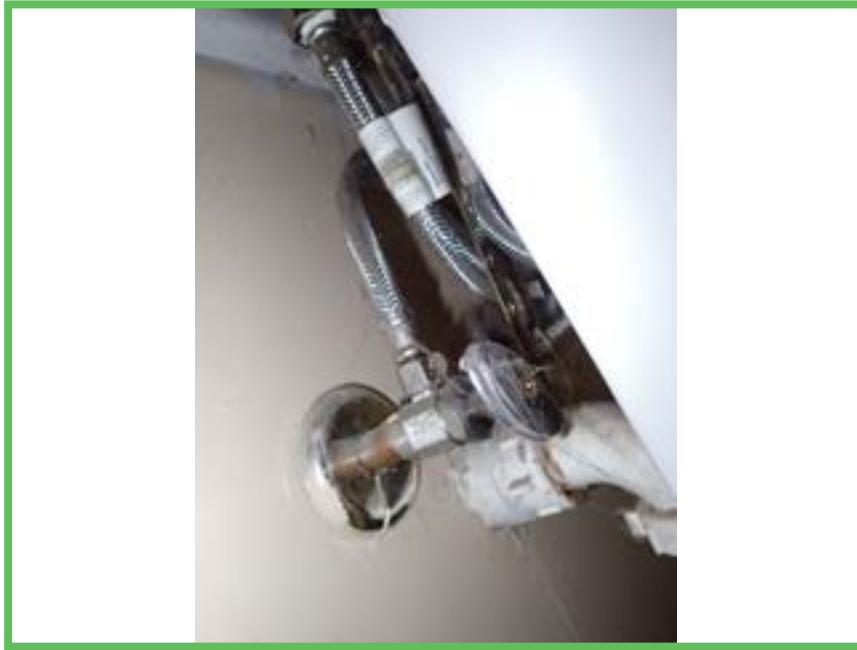
Under Sink1 Bath 1
