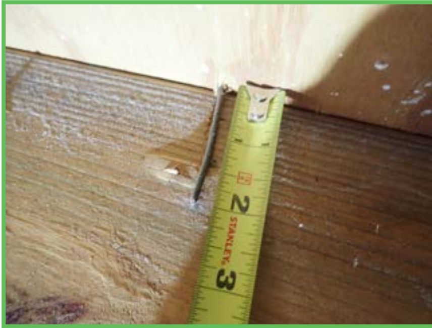
Roof Deck Attachment
