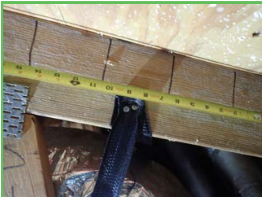
Roof Deck Attachment
