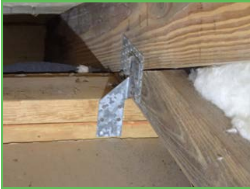
Roof to Wall Attachment
