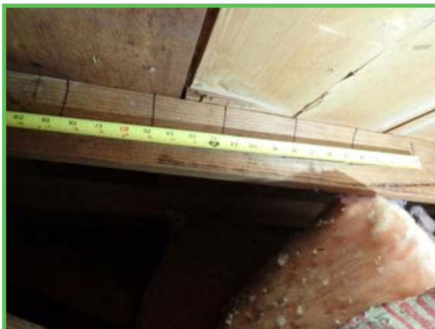
Roof Deck Attachment
