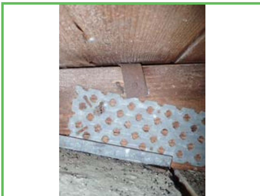
Roof to Wall Attachment
