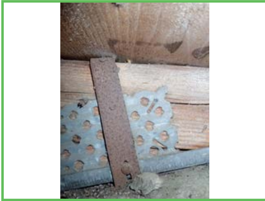
Roof to Wall Attachment
