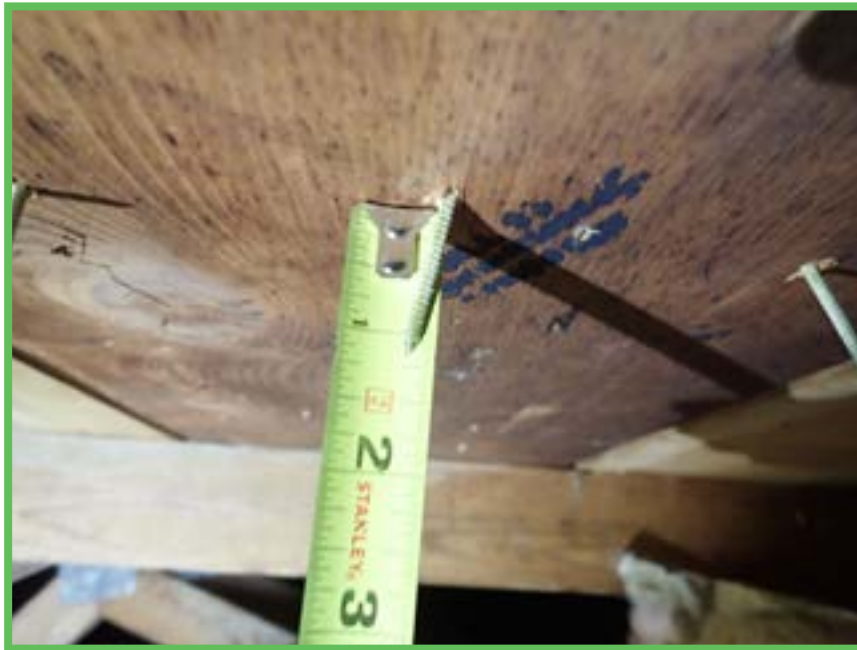
Roof Deck Attachment
