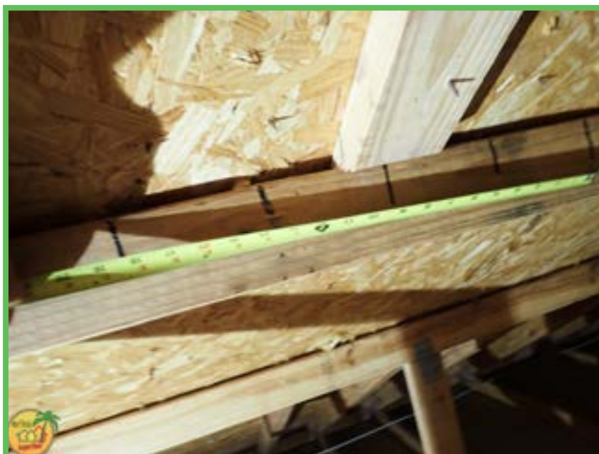
Roof Deck Attachment
