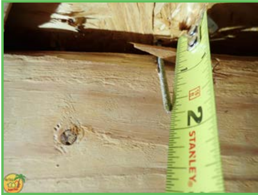
Roof Deck Attachment
