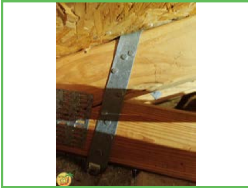
Roof to Wall Attachment
