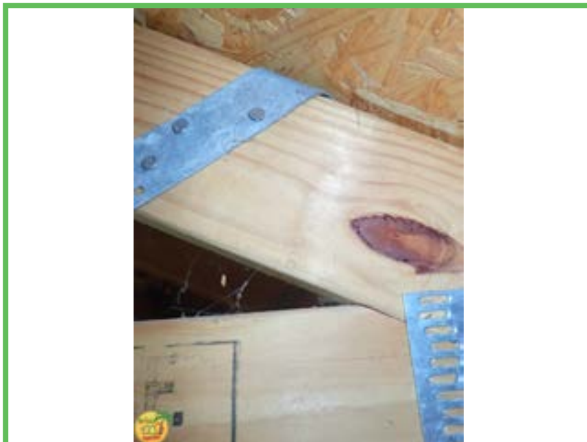
Roof to Wall Attachment
