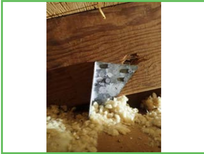
Roof to Wall Attachment
