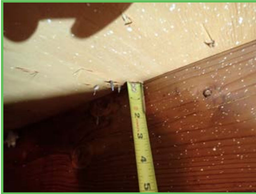
Roof Deck Attachment
