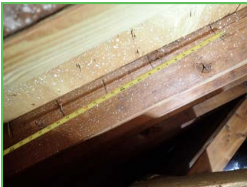
Roof Deck Attachment
