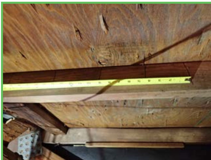
Roof Deck Attachment
