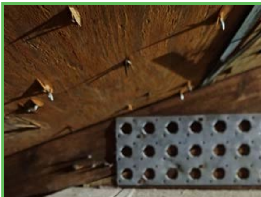
Roof to Wall Attachment
