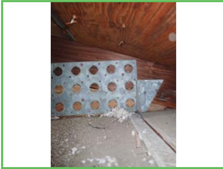
Roof to Wall Attachment
