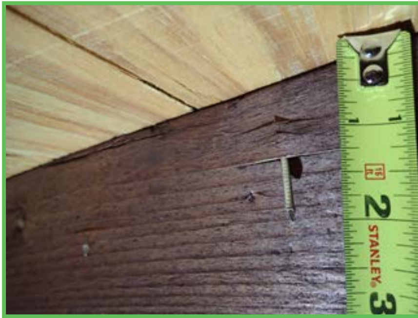
Roof Deck Attachment
