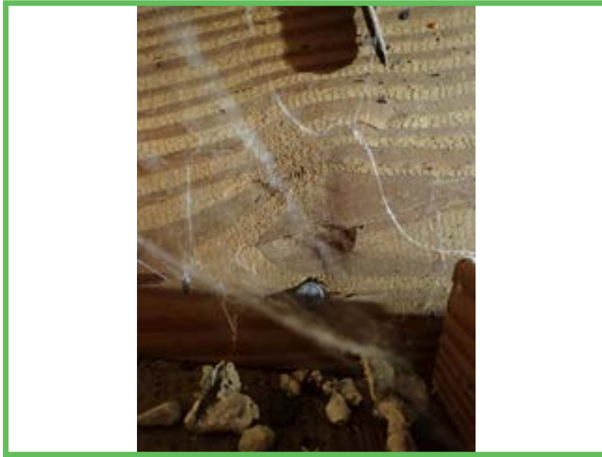
Roof to Wall Attachment
