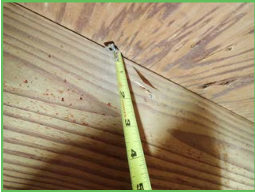
Roof Deck Attachment
