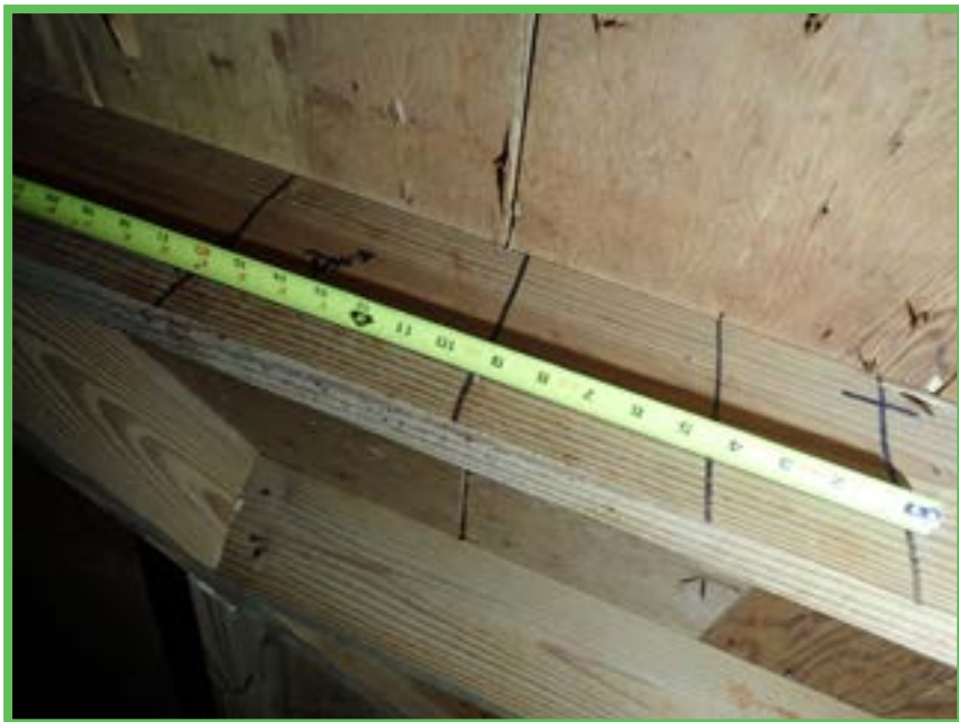
Roof Deck Attachment
