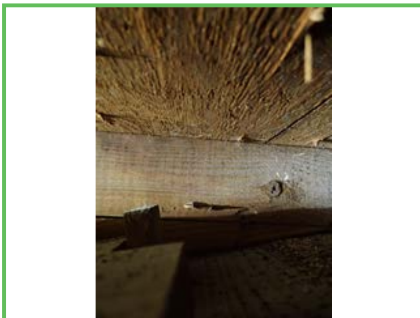
Roof to Wall Attachment
