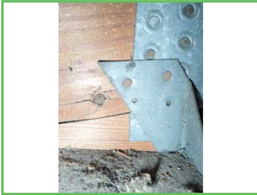
Roof to Wall Attachment
