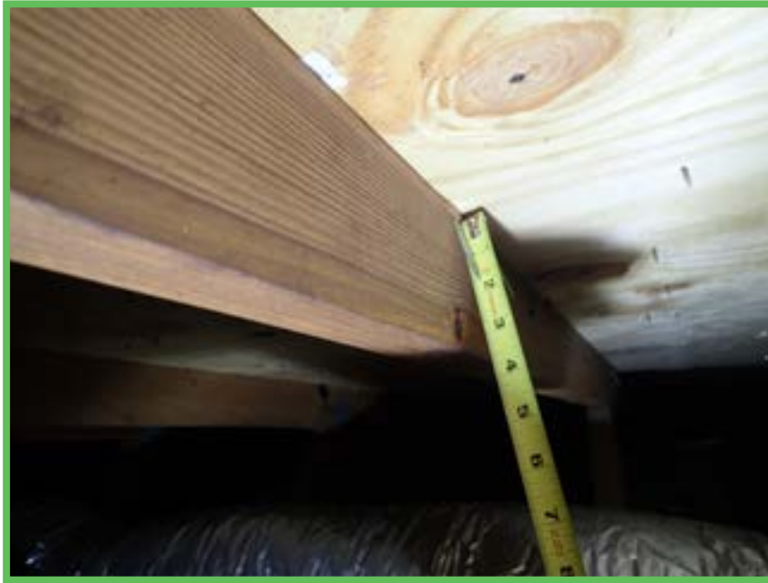
Roof Deck Attachment
