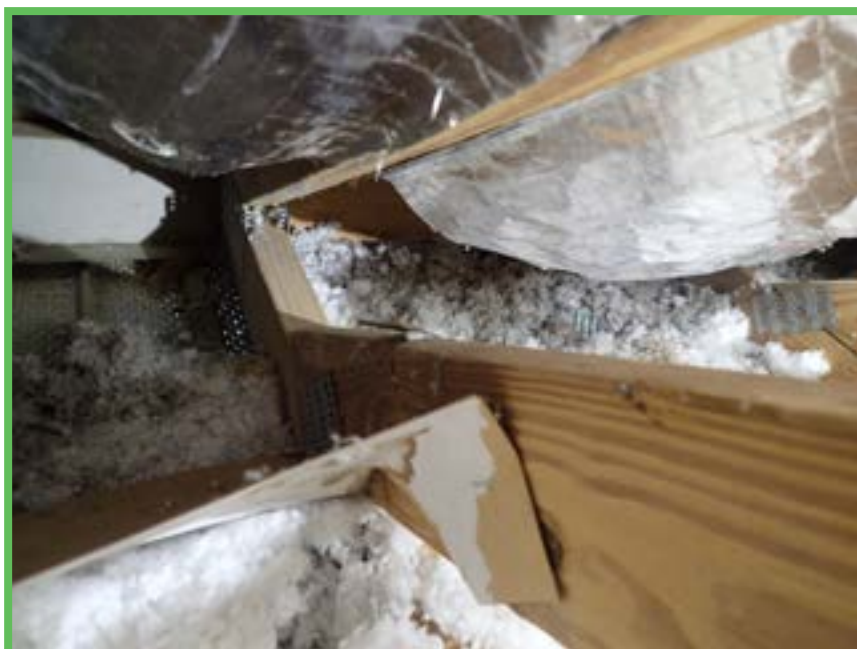
Roof to Wall Attachment
