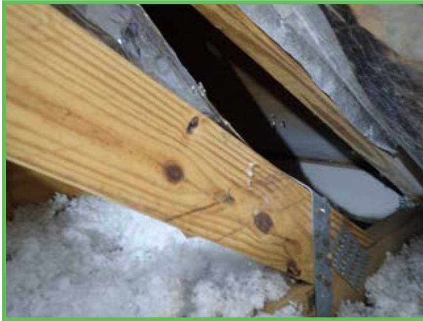
Roof to Wall Attachment
