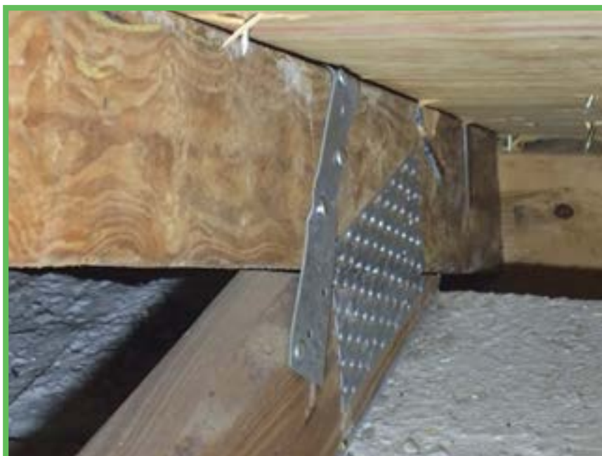
Roof to Wall Attachment
