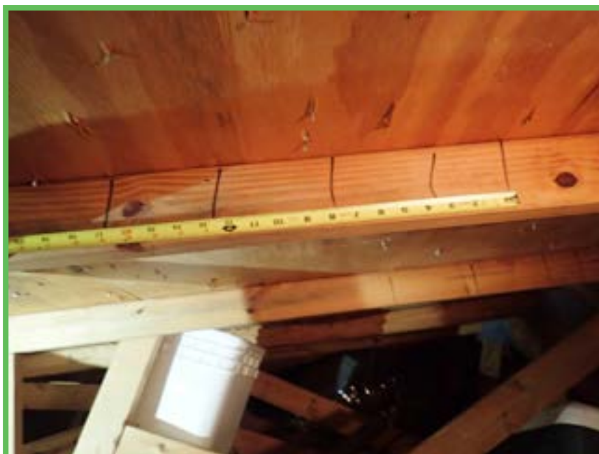
Roof Deck Attachment
