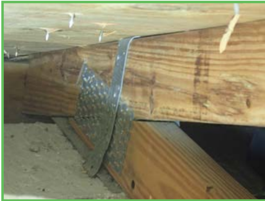
Roof to Wall Attachment
