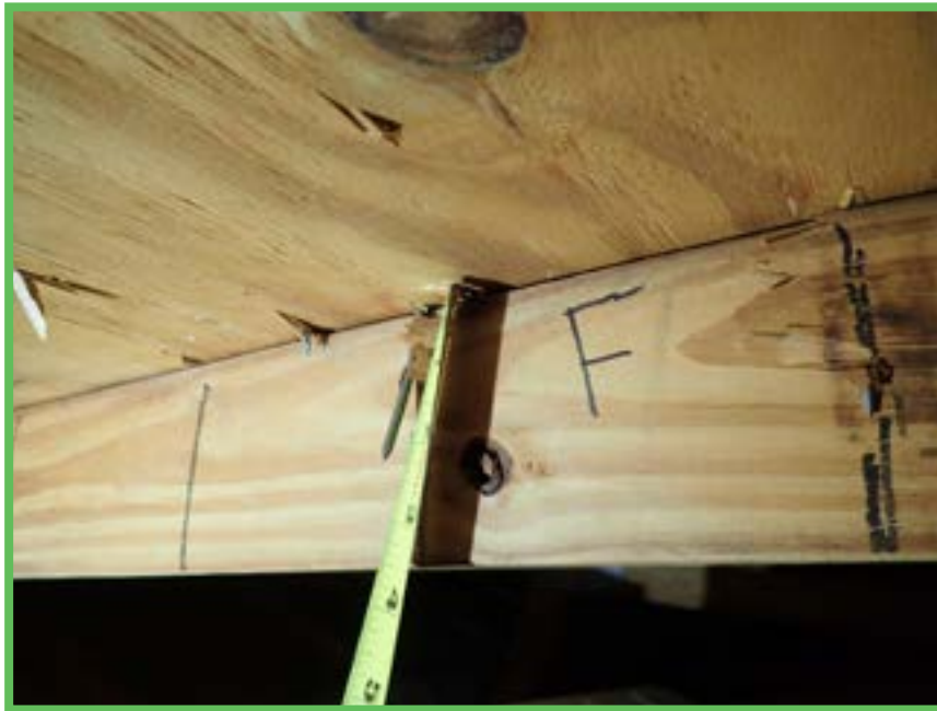
Roof Deck Attachment
