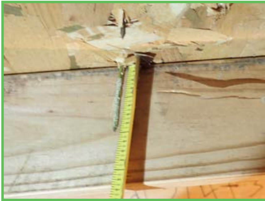
Roof Deck Attachment
