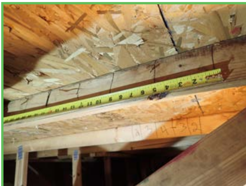
Roof Deck Attachment
