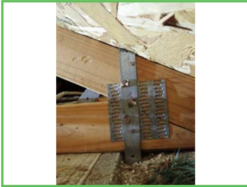
Roof to Wall Attachment
