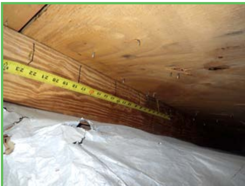
Roof Deck Attachment
