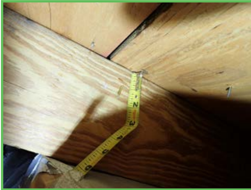
Roof Deck Attachment
