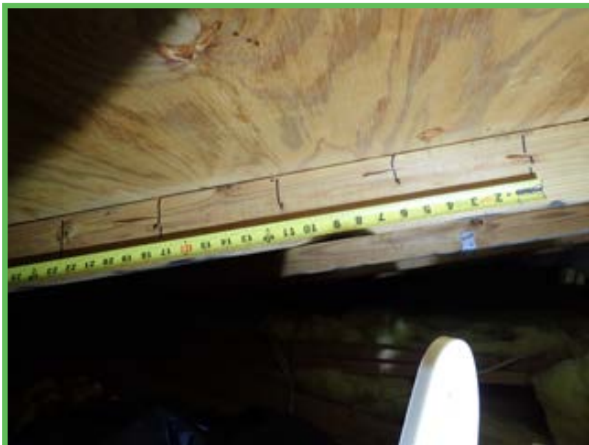
Roof Deck Attachment
