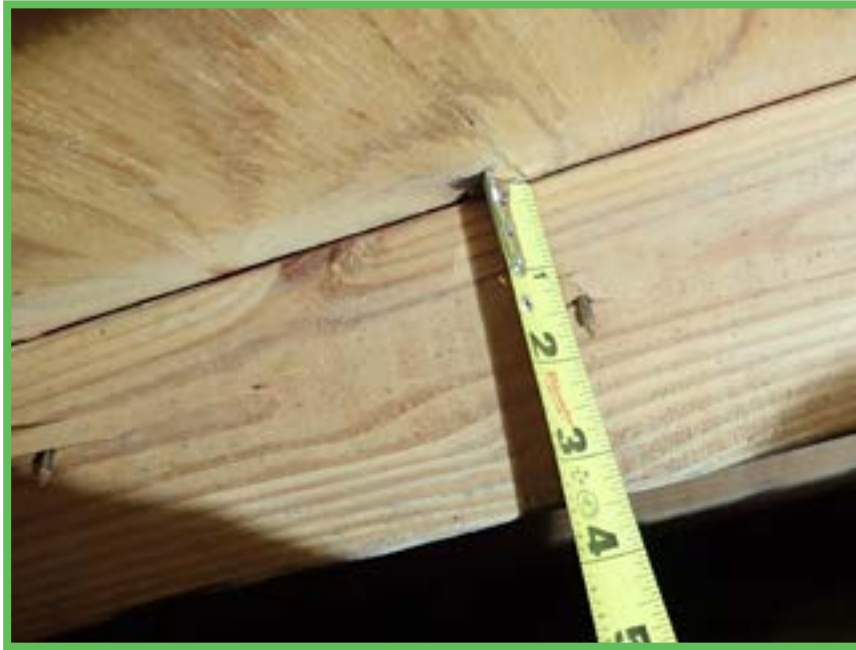
Roof Deck Attachment
