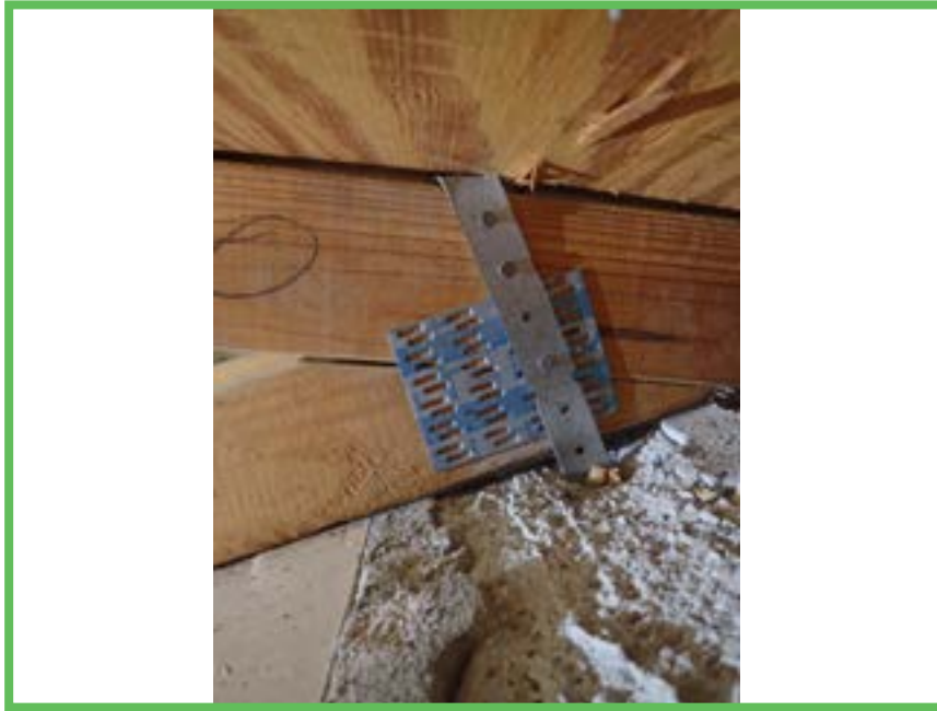
Roof to Wall Attachment
