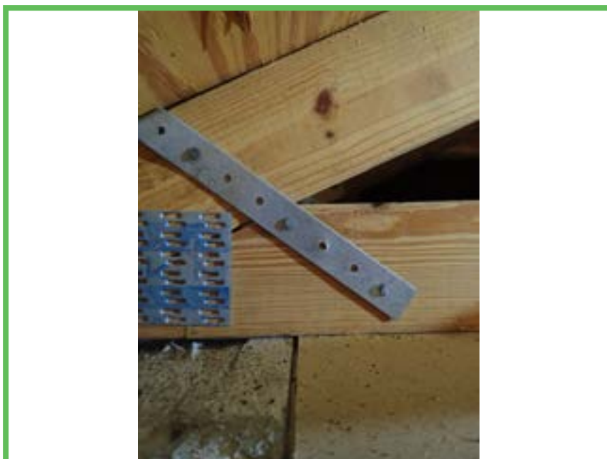
Roof to Wall Attachment
