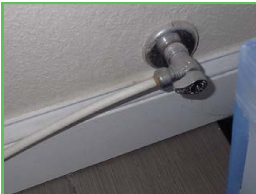
Master Bath Toilet Valve
